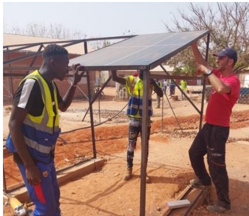
PV module installation
