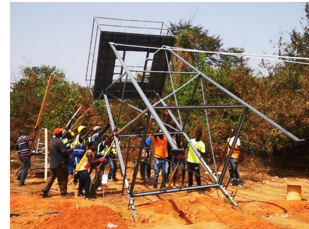
Water tank frame assembly
